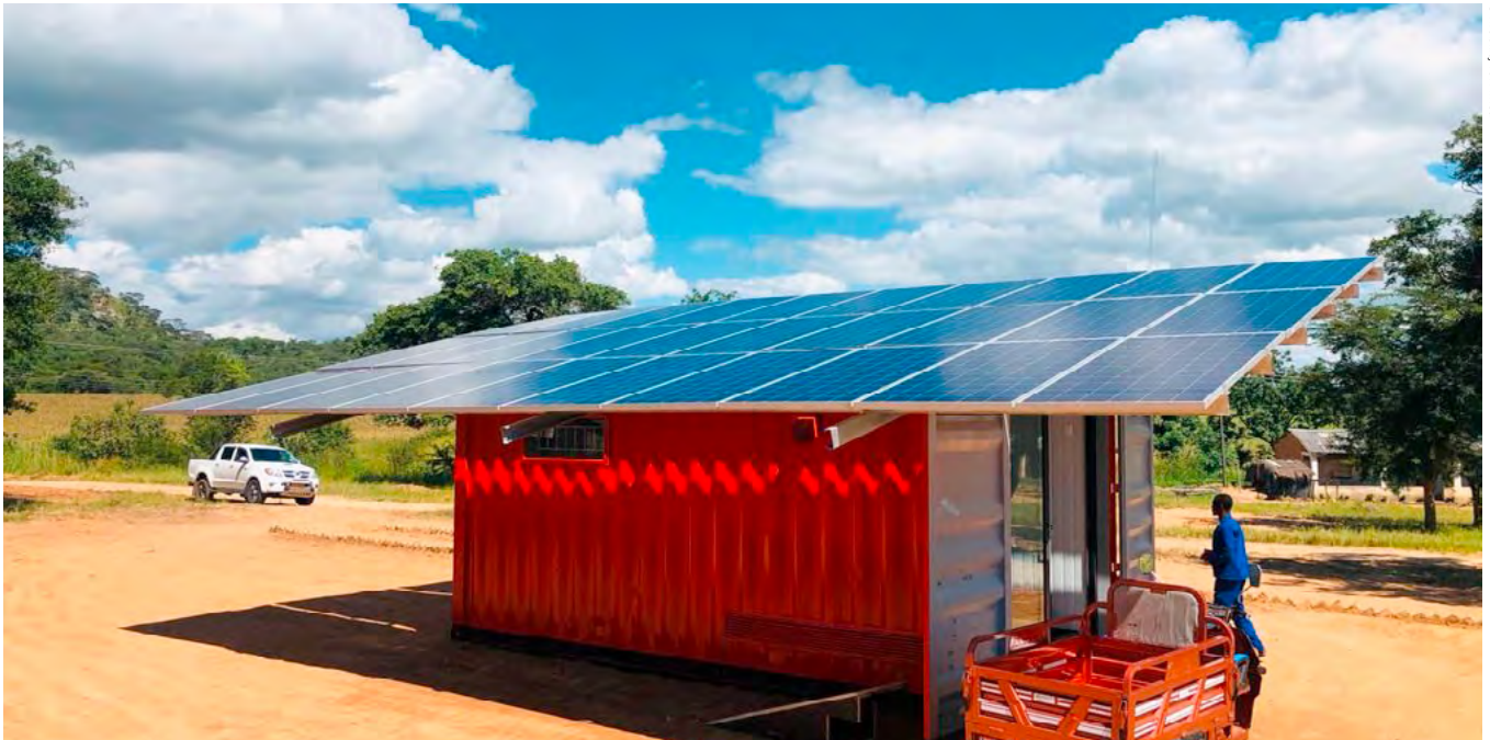
A community based solar charging station installed by MFA help charge the e-tricycle batteries in off-grid conditions (Zimbabwe 2019)
