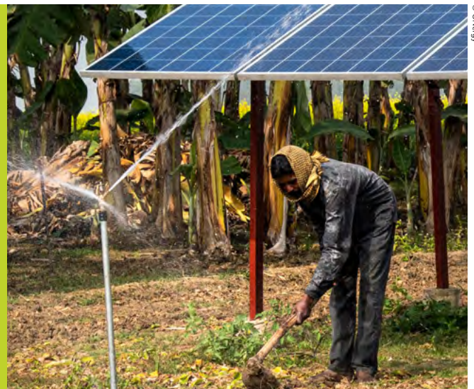
Micro-irrigation systems such as sprinklers attached with ONergy Solar Pumps are integral for climate smart agriculture (West Bengal, 2020)
