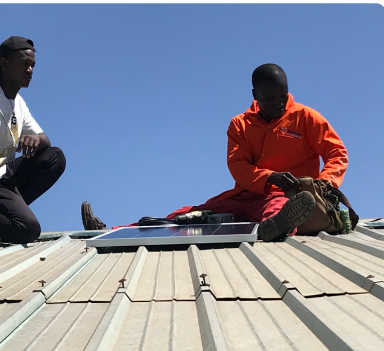
Installation of photovoltaic panels
