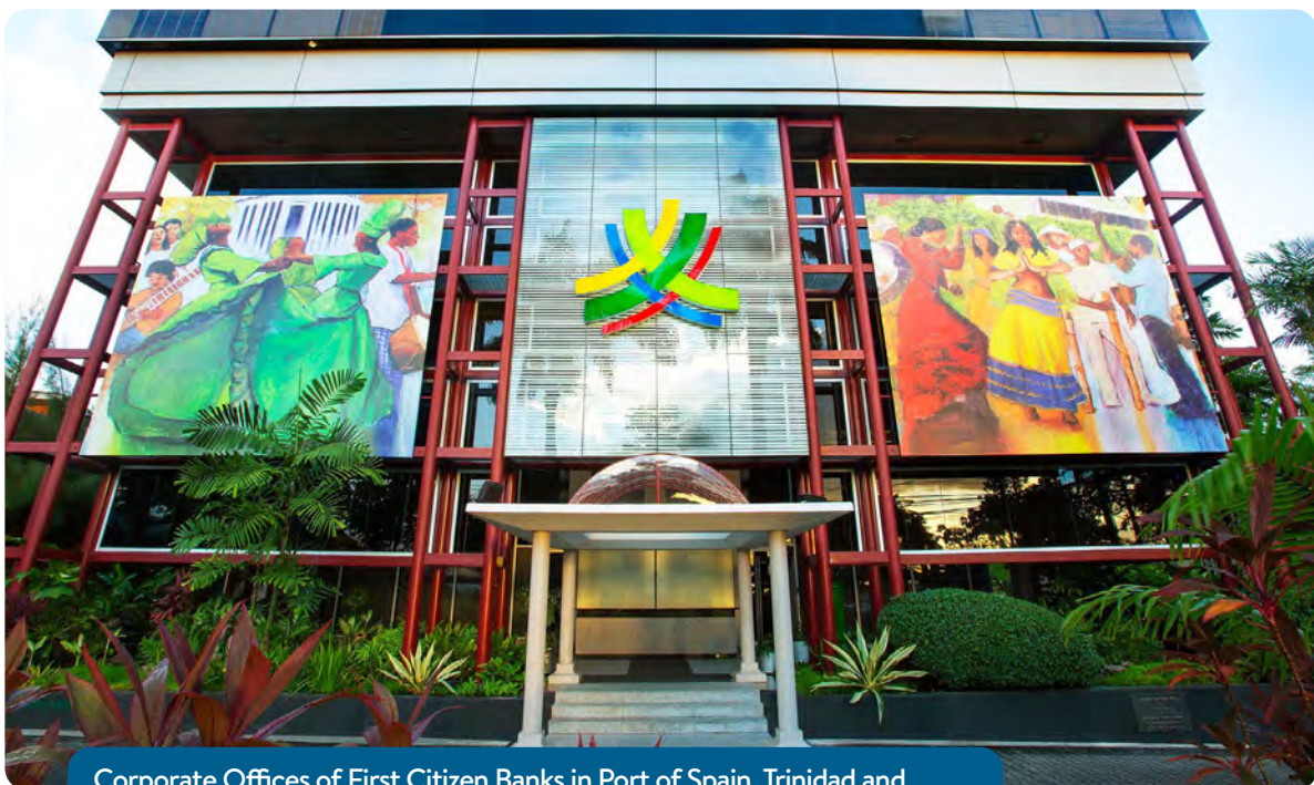
Corporate Offices of First Citizen Banks in Port of Spain, Trinidad and Tobago. Credit: Antony Scully/Scully Photography
